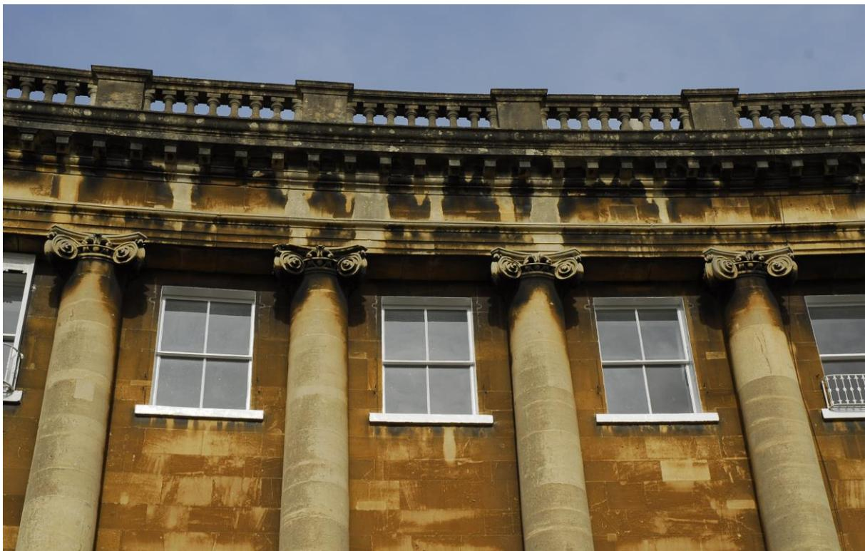
Figure 3 Detail of weathering pattern to elevation
