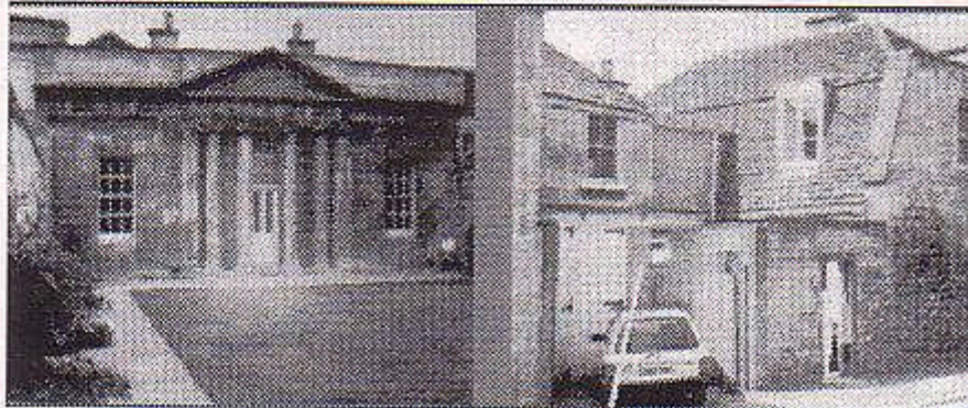
The coach-house at No 13 looks like a Greek temple from the garden view, left, but has a simpler elevation from its Crescent Lane entrance, right.
